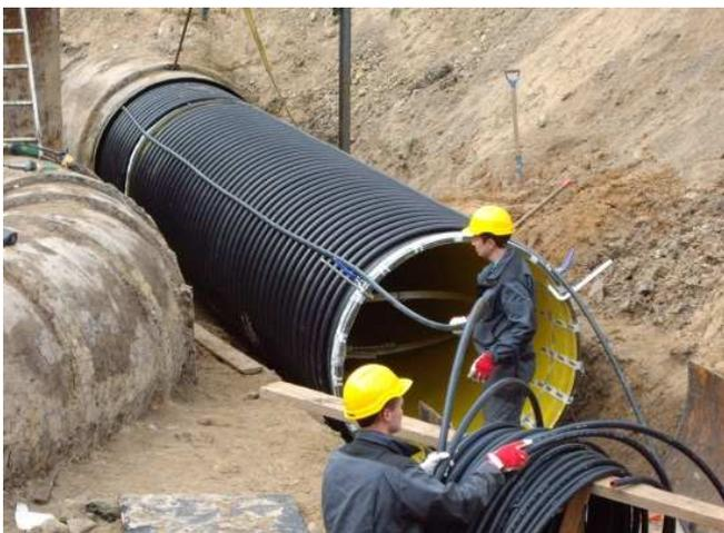
Image 6 - Start point of the relining, Krah electro-fusion welding and bentonite pipe installation
