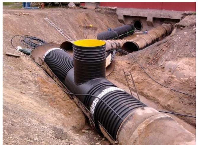
Image4 - E-fusion connected pipe with integrated pressure manhole to the main pipeline
