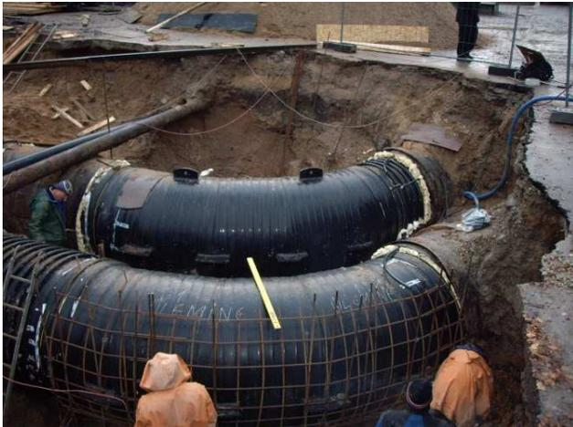
Image 8 - Preparing of the 60 degree bends for concret supports
