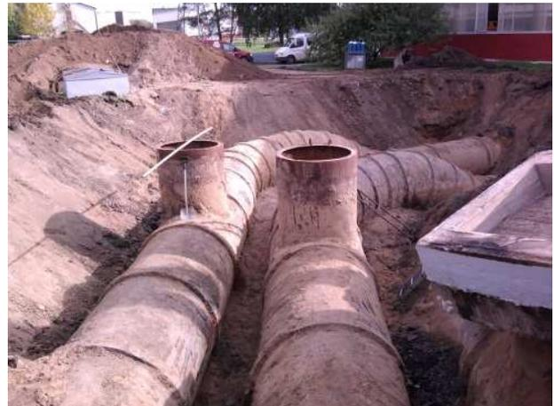
Image 1 - Original pipelines exposed
