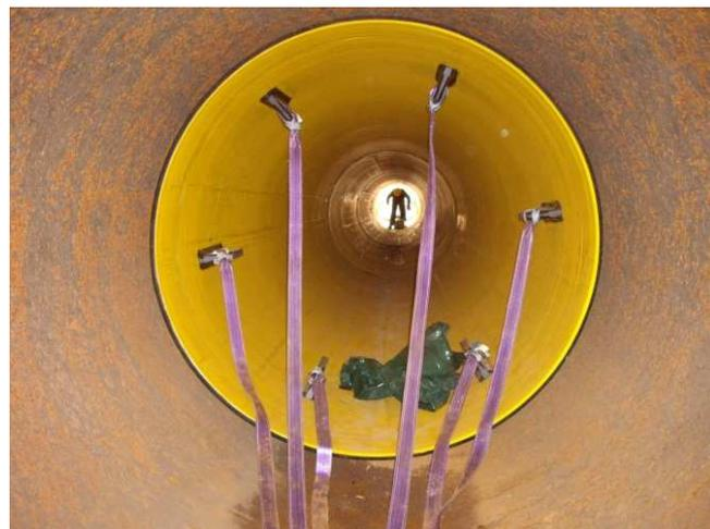
Image 7 - Stubs for anchoring the pulling ropes and spreading pulling loads
