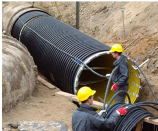
The original metal pipes had an inside diameter (ID) of 1580mm and wall thickness of 10mm. However, due to the smoother inner surface offered by BorSafe HE3490-LS, and therefore lower roughness coefficient than metal, calculations made by Tallinn Technical University determined that the corroded pipe could be replaced by pipe
